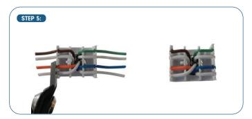
Cut the wires flush with the outside edge of the wire retention cap.
