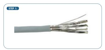
Remove approximately 50mm of the cable sheath and separate the 4 pairs.
